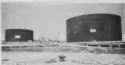
New Kero-Jet Fuel tanks. (Tankinano nobo pa Kero-Jet Fuels).
